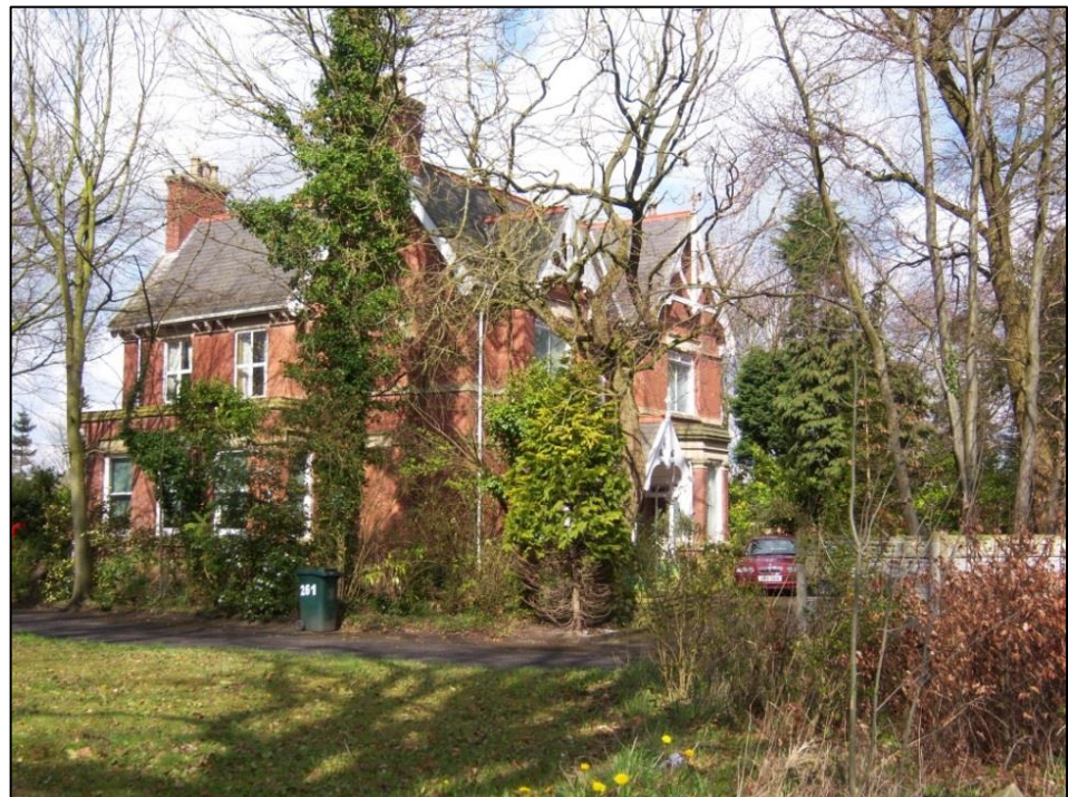
Clayton House, Liverpool Road South
