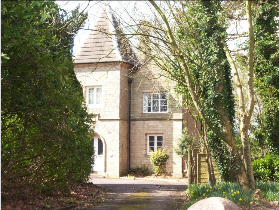
255 Liverpool Road South
